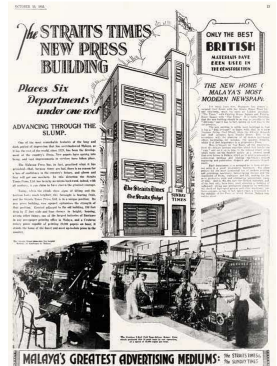
The Straits Times announcing the completion of its new building on Cecil Street in 1933. Designed by Doucham Petrovitch, it marked Swan & Maclaren's return to Modernism after its first foray with the St Andrew's Mission Hospital a decade earlier. The Straits Times , 10 October 1933, p. 17.
