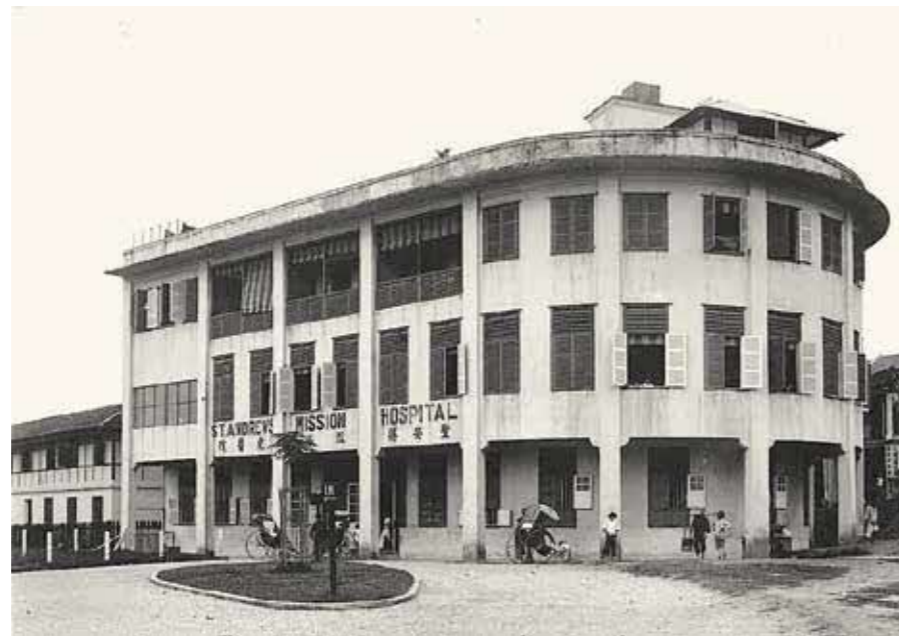
St Andrew's Mission Hospital at Erskine Hill, photographed in 1938. Designed in 1922 by Harry Robinson of Swan & Maclaren, the three-storey concrete frame building provided accommodation for 50 in-patients with additional quarters for the European and Asian staff on the top floor. The flat roof afforded recreational space for both staff and patients. Courtesy of St Andrew's Mission Hospital.
